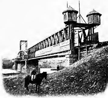
GATES READY TO BE SHUT AGAINST THE CONFED- ERATES
